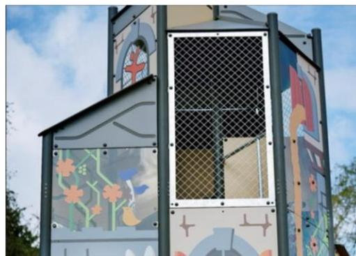
Fully welded steel frame with 45° cross welded steel grid of round steel pins with a diameter of 4mm. The airflow panel contributes to the overall structural integrity of the GIANT towers.
